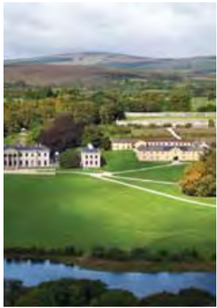
The Picnic House is situated within Ballyfin's grounds, close to the main house
