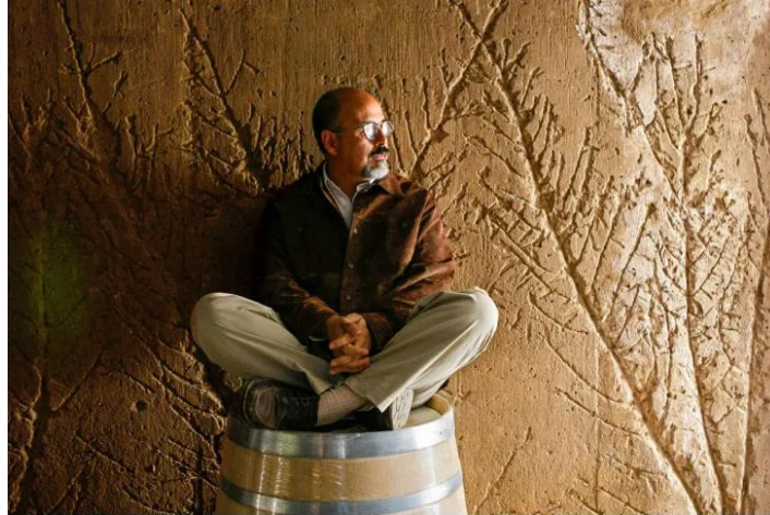
D'ACOSTA AT PARALELO, WHERE FRESH OLIVE BRANCHES WERE USED TO LEAVE DECORATIVE IMPRESSIONS IN THE RAMMED EARTH WALLS / IMAGE COURTESY OF DON BARTLETTI
