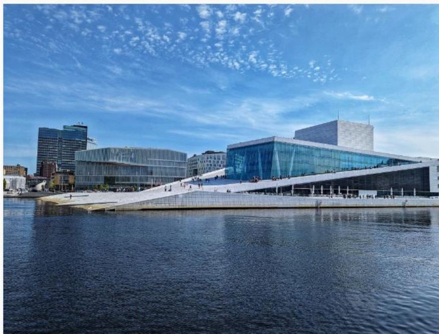
The Oslo Opera House
